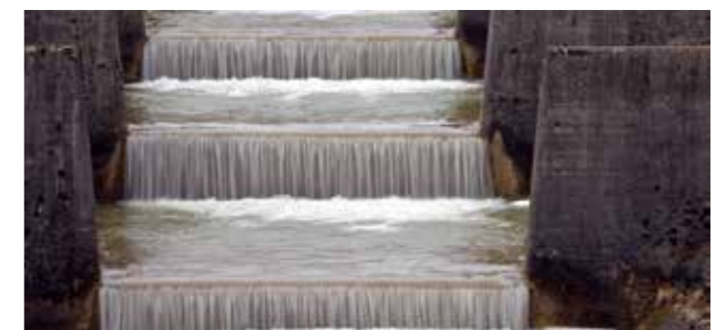
Particularly in whitewater, concrete surfaces are subject to massive additional strains by rubble, sharp edges and abrasion, as well as possible temperature stresses due to frost exposure.
