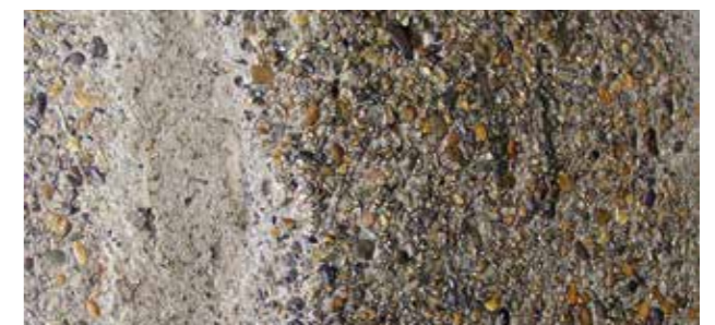
Due to continuous exposure, the cement film is eroded in an initial step, and thereafter larger and larger aggregates are rubbed, knocked or washed out of the hardened cement paste
