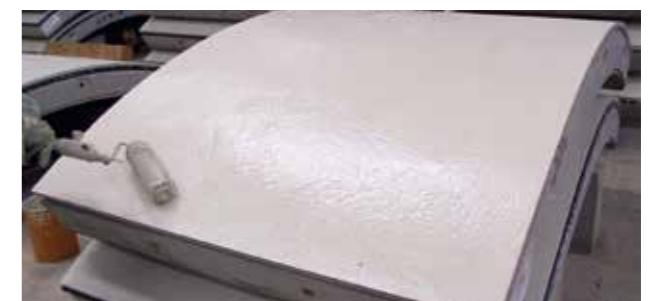
Immediately following curing in a steam channel, the concrete surface of tunnel lining segments is coated with water-based epoxy emulsion that is absorbed even into the smallest pores, thereby generating a sealed, protective coating.
