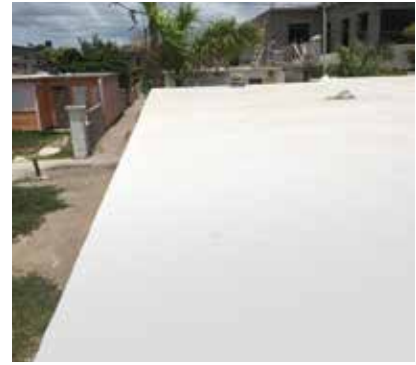
Finished roof with 3 coats of Sikalastic®-560.
