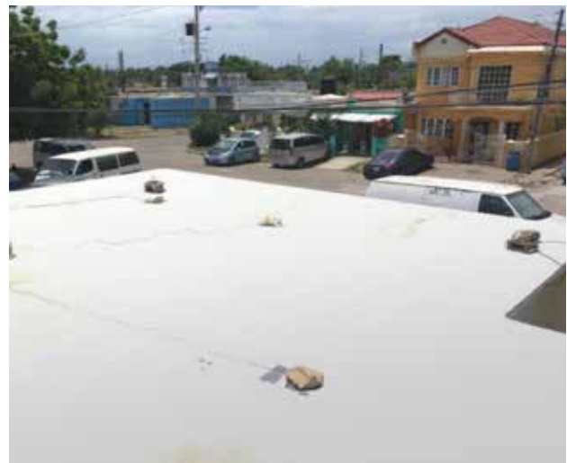
Roof after the application.
