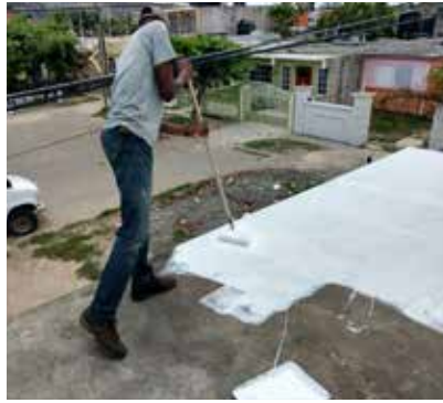
Application of Sikalastic®-560 diluted with 10% water as a primer.
