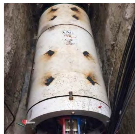
Owner: ADREW Alger Project management: COSIDER M35 Control laboratory: Technical Hydraulic Control Design Office: CTH
