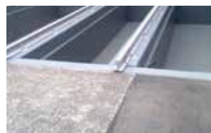
Solutions for Secondary Containment Areas. Page 40
