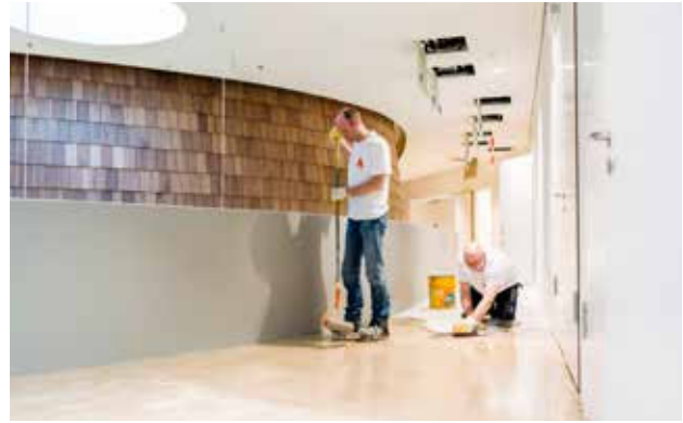
STEP 2. A liquid primer is applied to assure good bonding of the flooring, which is typically done by trowel and roller. The adequate method can be selected depending on the quality of the subfloor.
