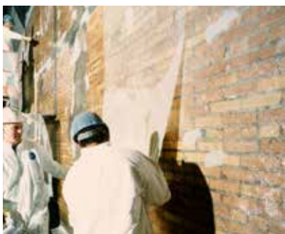
SEISMIC UPGRADING /EARTHQUAKE DAMAGE REPAIR
