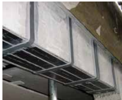
BEAM STRENGTHENING
