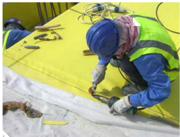
6 Compartmentalized sheet membrane systems
