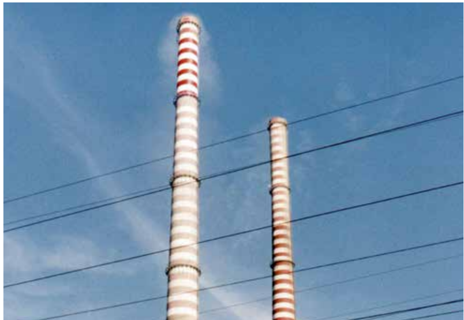
Chimneys in direct sunlight indicating variations in thermal exposure which are further exacerbated by the effects of the downward flow of hot exhaust gases during periods of temperature inversions.
