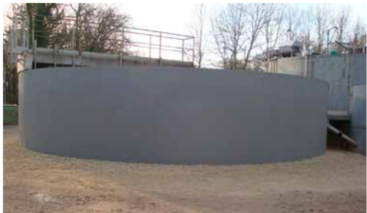
Completed work, not a day's interruption.
