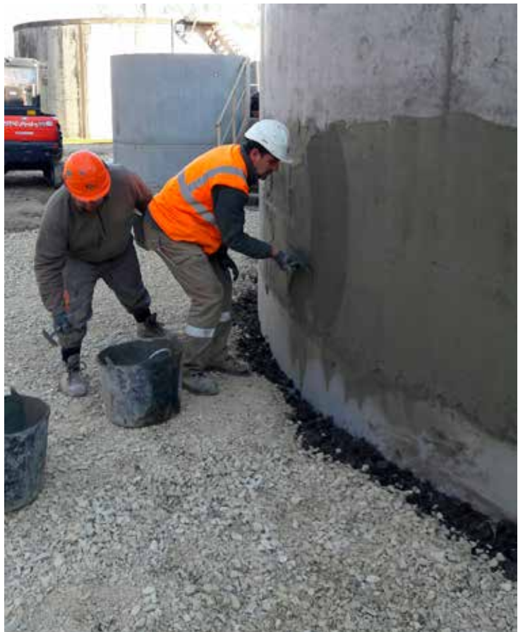
Implementation of the system without interrupting the structure.
